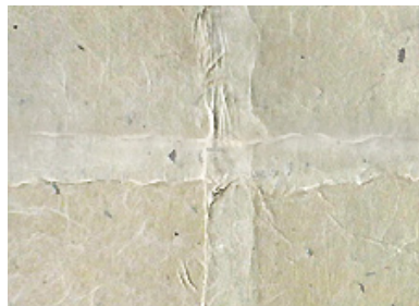
overlap installation (live edge)
